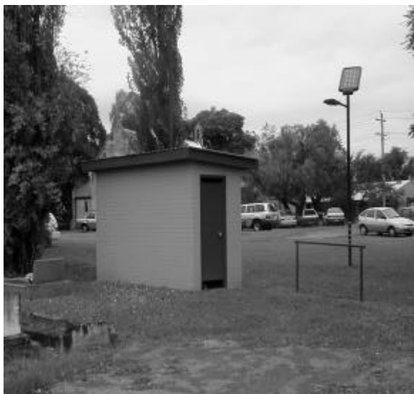
Emu Plains toilet block and solar light
